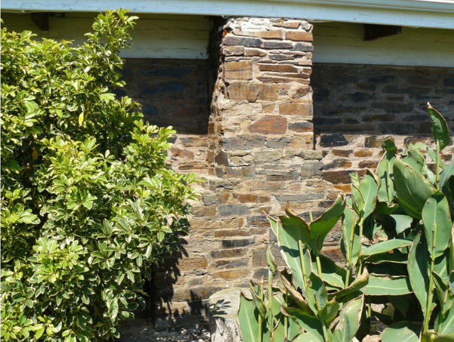
Plate 5 An original external stone chimney.
