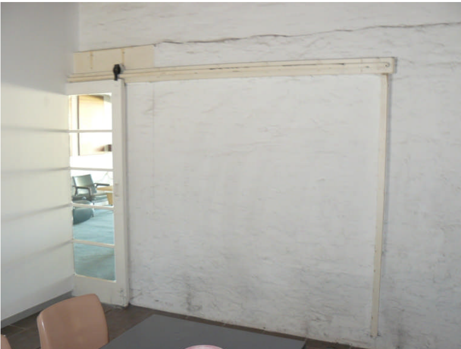
Plate 4 An original painted metal sliding door.
