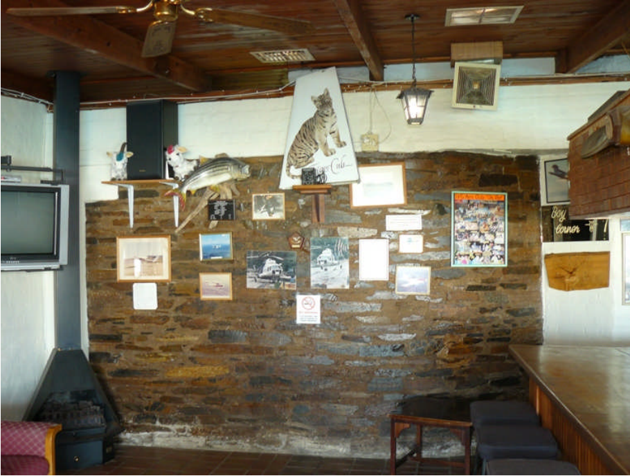
Plate 3 An original external wall, enclosed by later extensions.
