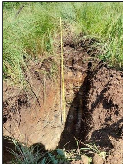
**Plates 9 & 10: Typical soil profiles encountered beneath the site; clayey residual soils overlying the generally shallow, completely to highly weathered shale rock of the Pietermaritzburg Formation**
