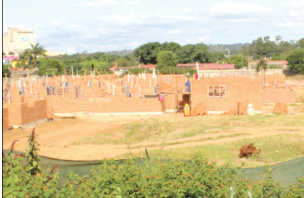
Construction at the Jika Joe Housing Project (Photo: Mbulelo Baloyi)
