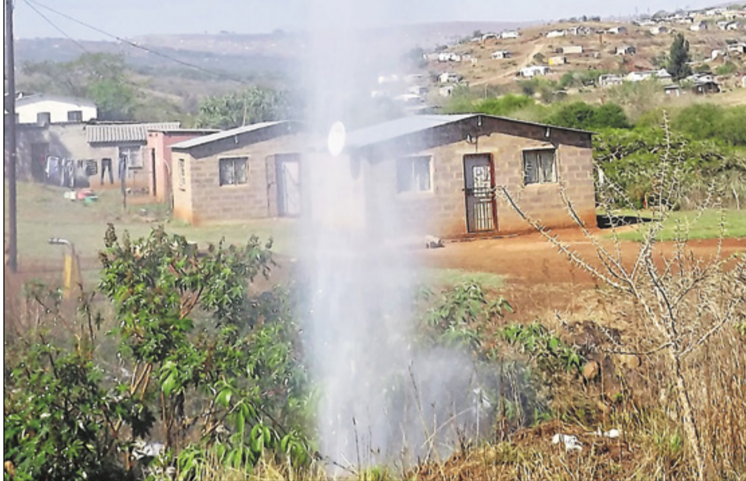
A broken communal standpipe causing concern (Photo: Nompandolo Ngubane)
