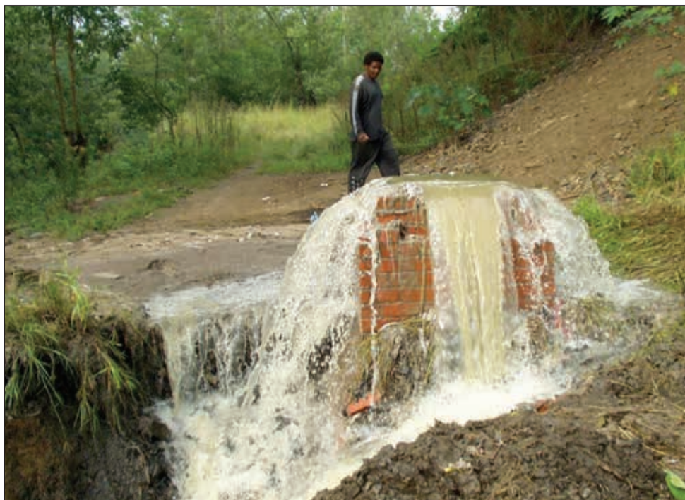
Overflowing sewer manholes and water leaks (Photos: DUCT / Ian Carbutt)
