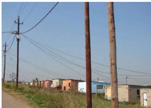
CINDERELLA PARK ELECTRIFICATION
