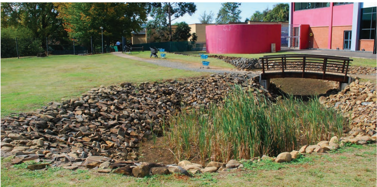
Figure 12: Bio-swale to enable stormwater filtration and infiltration (KZN)
