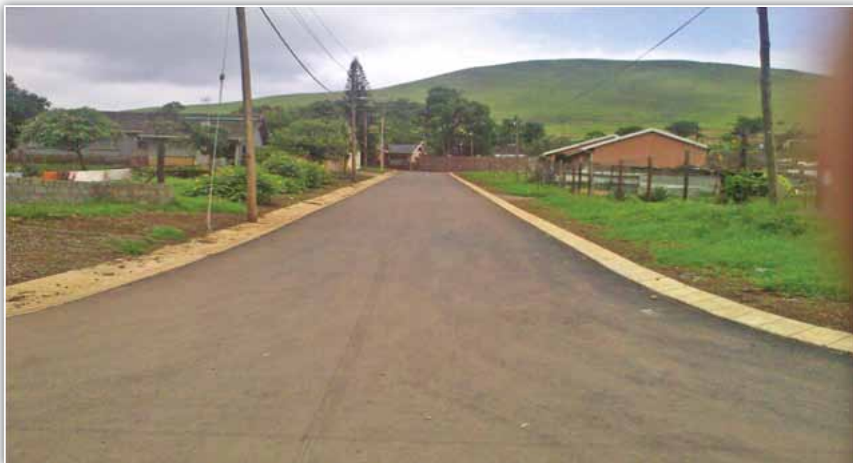
ABOVE: Harry Gwala Road in Dambuza
