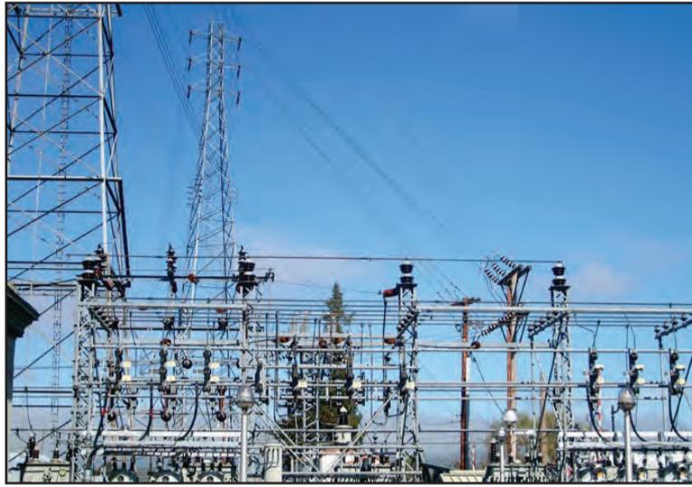
One of the power stations that ensures the stable supply of electricity to households and industries in the city.
