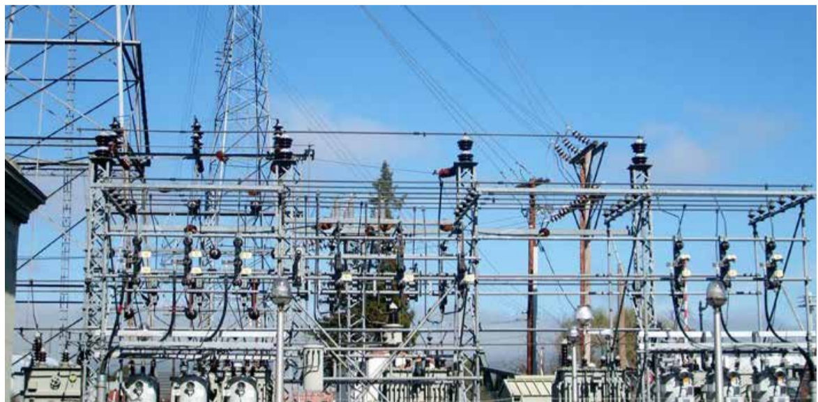
Stable power supply is an important component in attracting business and investment, and this is one of the reasons that Msunduzi Municipality is upgrading power stations in different parts of the municipality.
