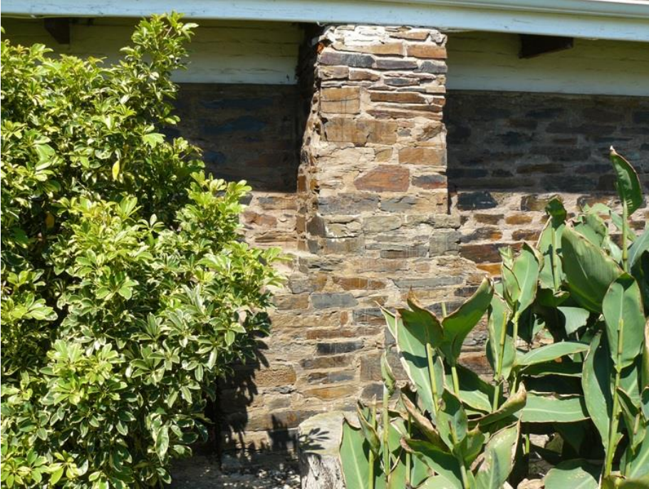
Plate 5 An original external stone chimney.
