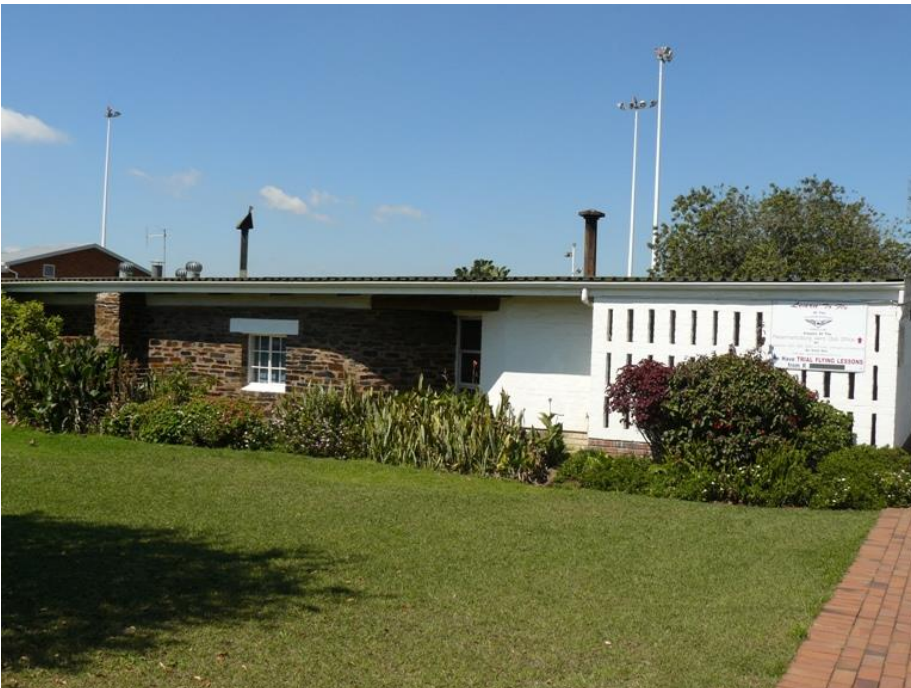
Plate 2 The north-western side of the original clubhouse building with extensions to the west.
