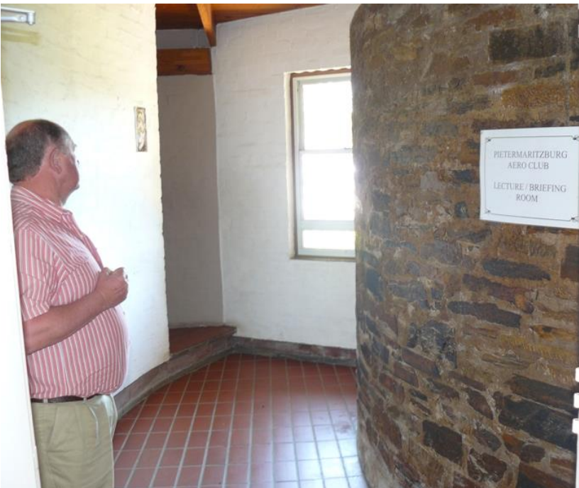
Plate 6 Mr Dave Campbell viewing an original stone exterior wall, now enclosed.
