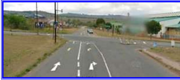
Market Road – Washington / Market Road Extension intersection
