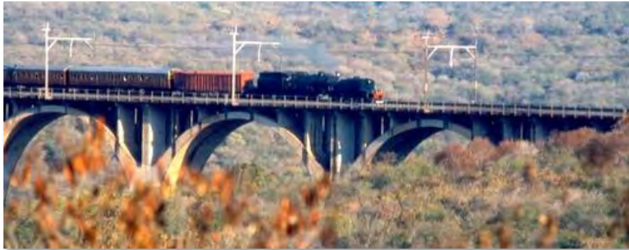
Figure 6: The Mkondeni Viaduct (Source: Google Earth)
