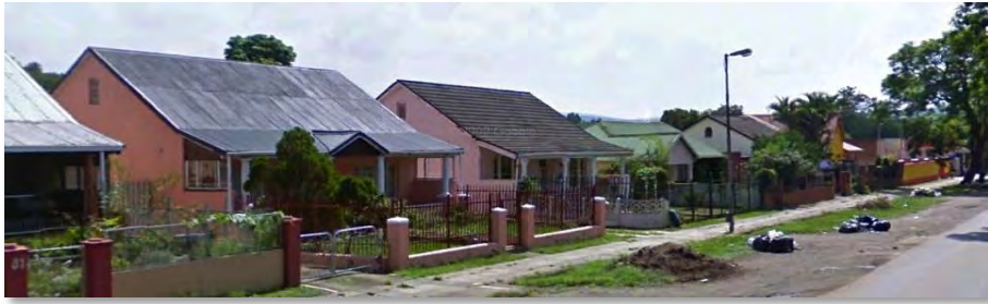
Figure 6: Built form character: lower density residential areas
