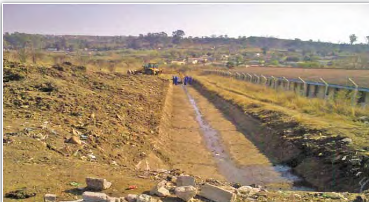
ABOVE: Storm water channel cleaned by Drainage Maintenance Team
