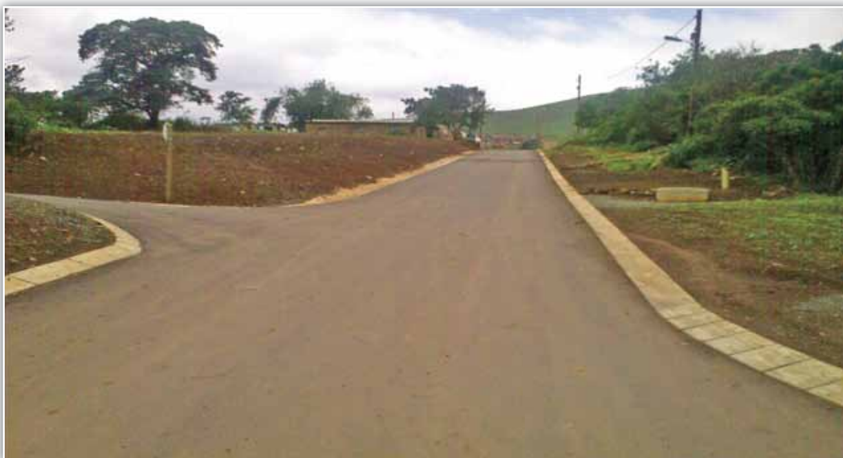
ABOVE: Machibisa, Dambuza Road Project
