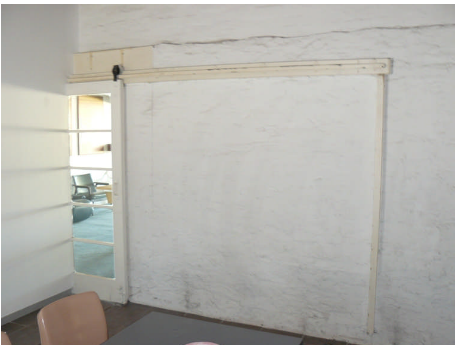
Plate 4 An original painted metal sliding door.
