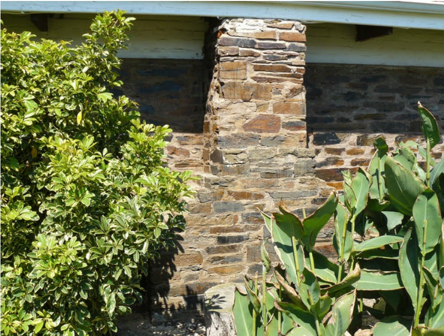
Plate 5 An original external stone chimney.
