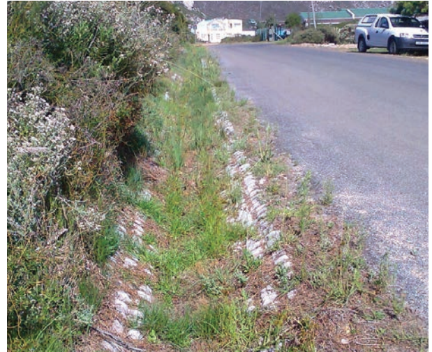
Figure 9: Bio-swale to enable stormwater filtration and infiltration (KZN)
