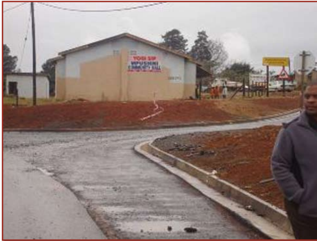
ROAD D1132 BEFORE CONSTRUCTION
