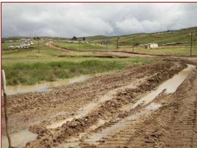
ROAD D1127 UNDER CONSTRUCTION
