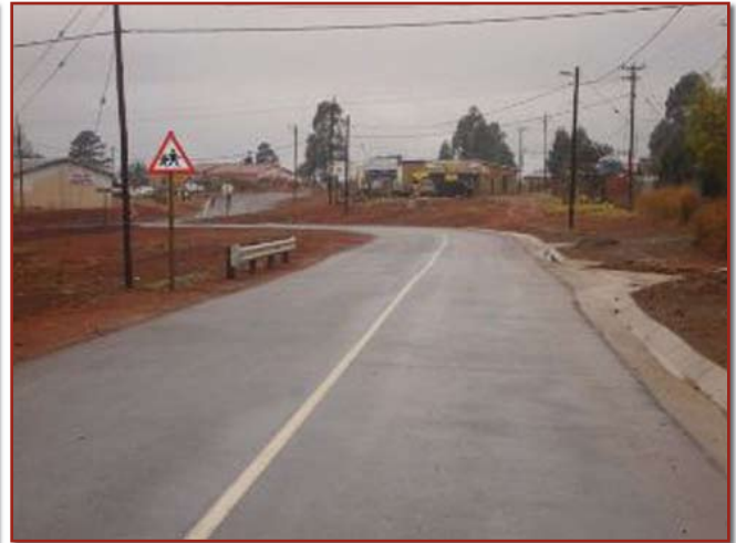
ROAD D1132 CONNECTING TO ROAD D1137 AFTER CONSTRUCTION
