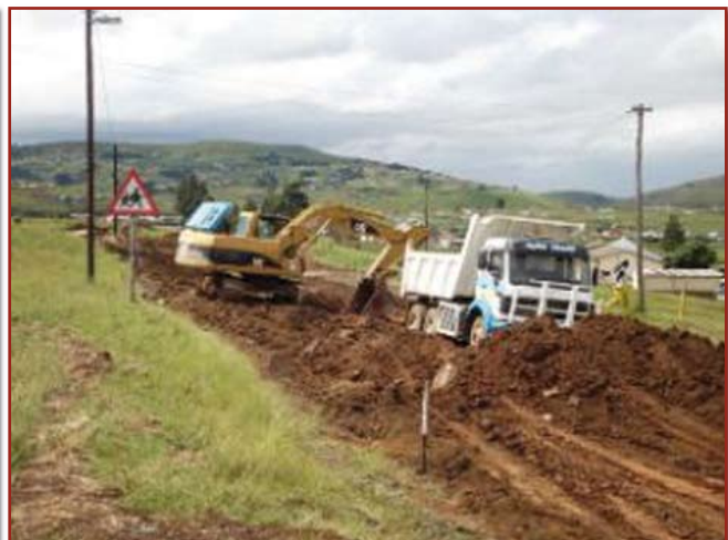
ROAD D1127 UNDER CONSTRUCTION
