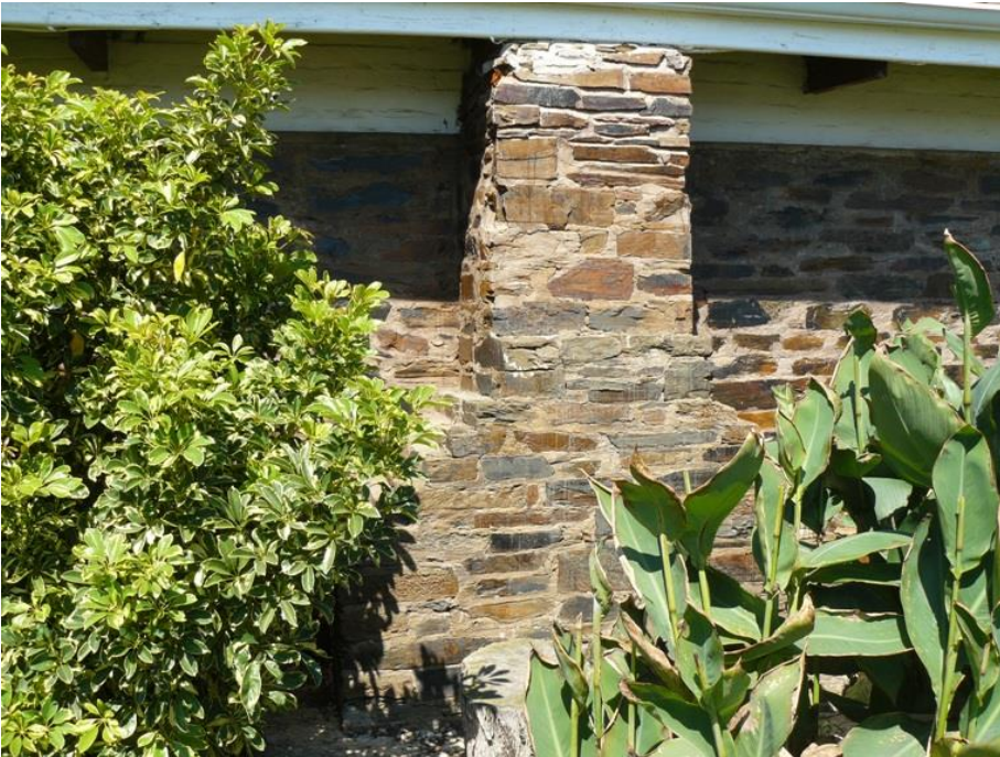
Plate 5 An original external stone chimney.
