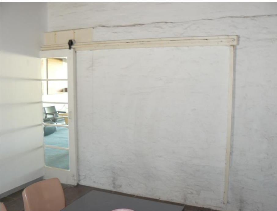
Plate 4 An original painted metal sliding door.
