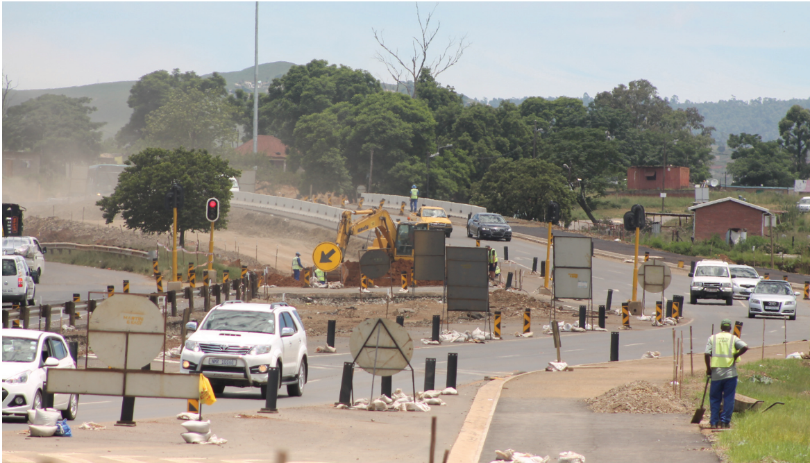
Kusaqhubeka ukwakha emgwaqweni u-Edendale Road okuyimanje uyandiswa ngaphansi kohlelo lwe-Integrated Rapid Transport Network okulindeleke ukuthi lwenze ukuhamba kwabagibeli kube lula.
