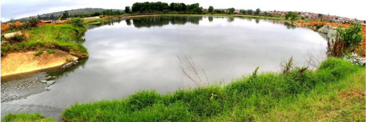
Figure 7. The lower dam showing the typically open-water nature of this waterbody and the largely exposed shorelines.
