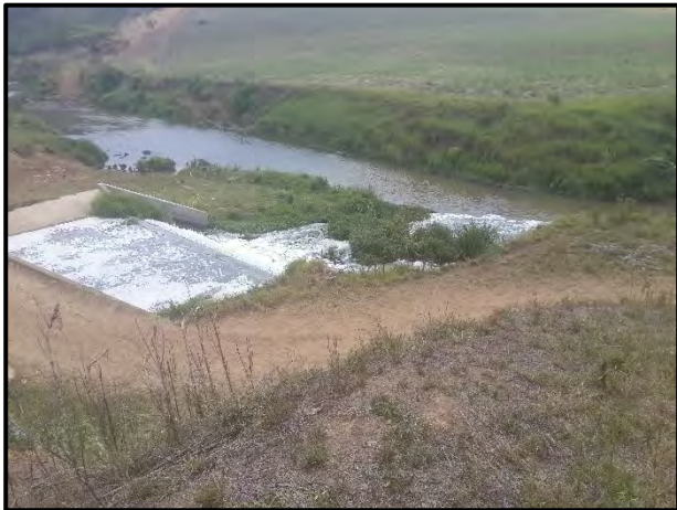
Plate 1: View of current treated effluent outflow from the Darvill Sewage Works into the Msunduzi River.
