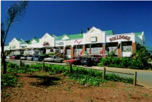
Commercial: Suburban Shopping Centre
