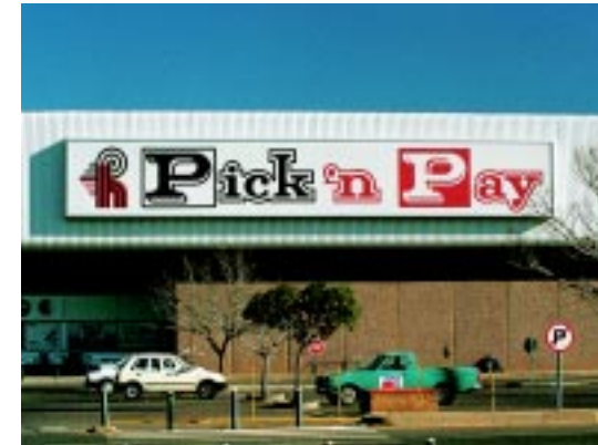
Commercial: Suburban Shopping Centre
