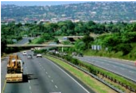
Transportation: Freeway, Pretoria
