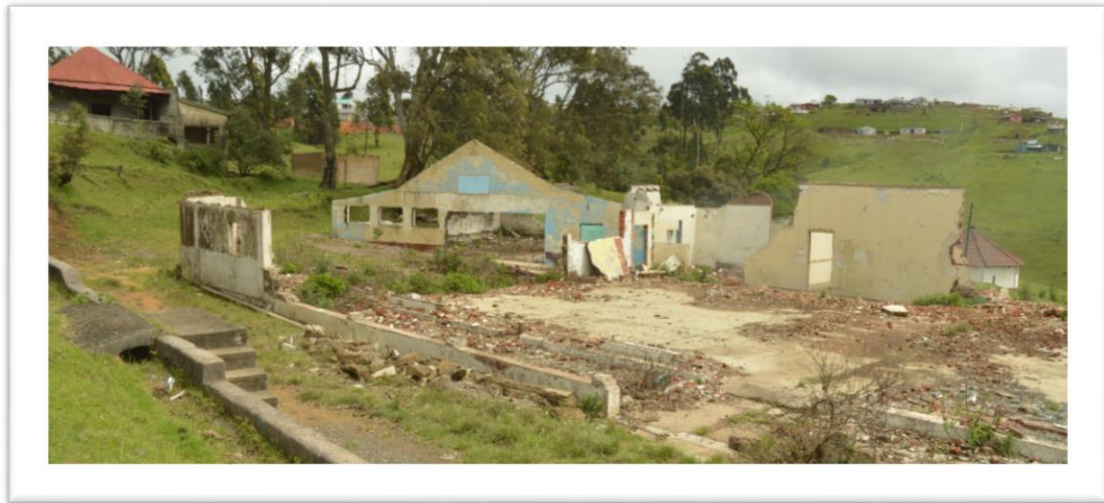
Figure 9: ex Petrol Filling Station and Motor Garage workshops north of Elandskop Station
