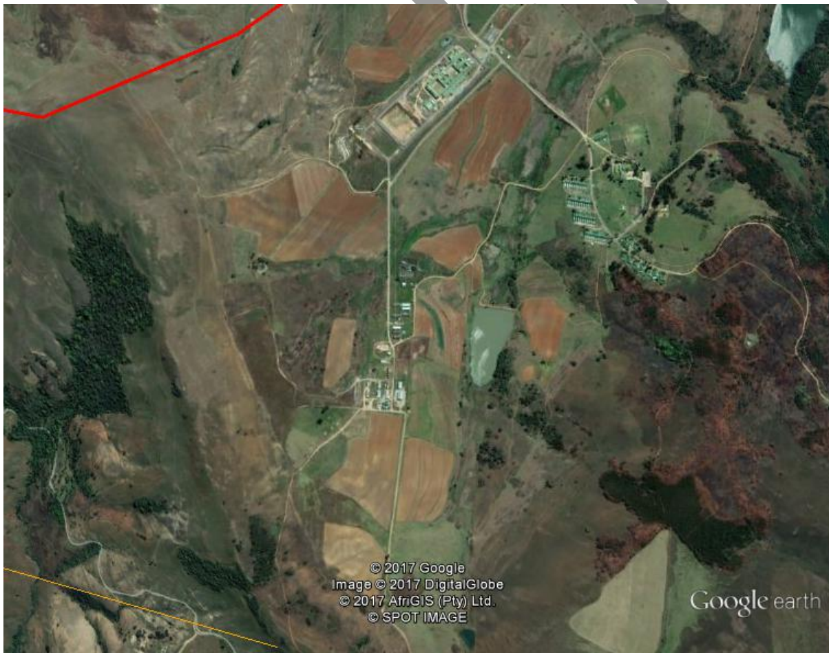
Photo 1: Land Use Severtfontein Correctional Facility (Google Earth, 2017)
