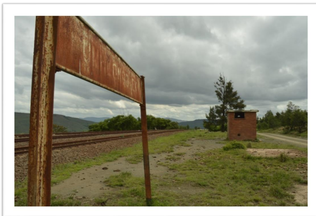
Figure 5: Umhlongonek Station remnants
