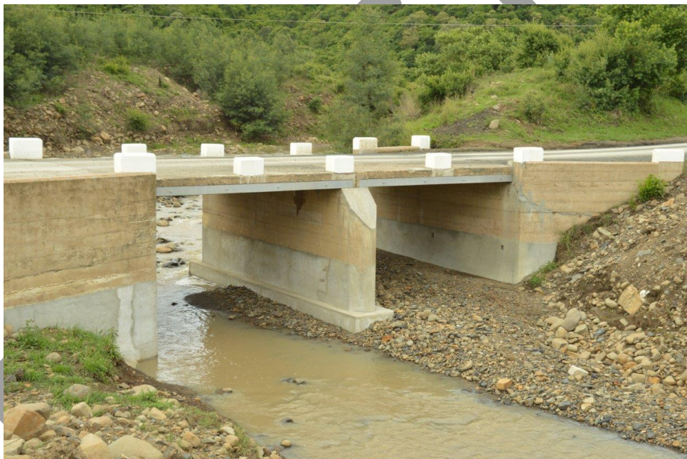
Figure 79: Recently (2017) partly re-constructed bridge of P121 over the Ncwadi River
