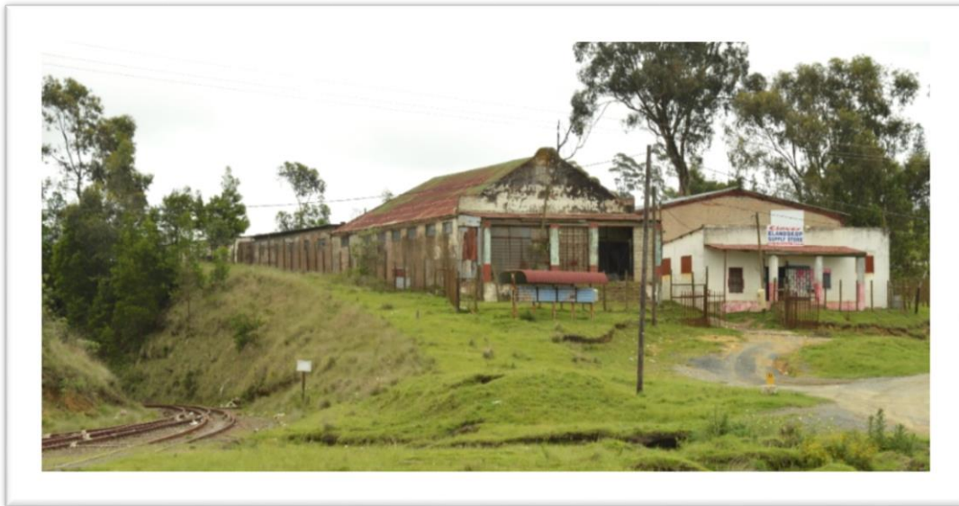
Figure 8: Ex-commercial and related buildings immediately west of Elandskop Station
