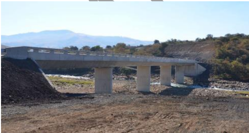
Figure 105: New bridge across Mkomazi River
